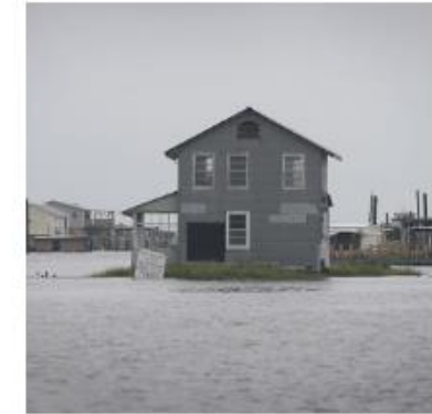
Storm Surge Hurricane Barry, Louisiana, 2019
